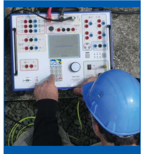
7. Operator using CBA 1000 in a substation test
